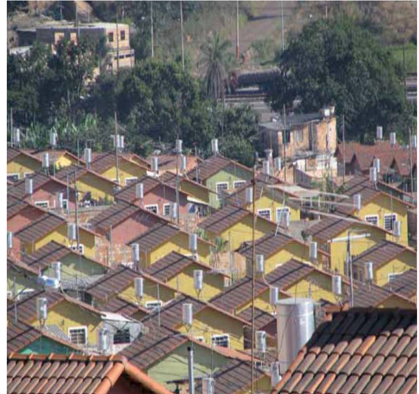
Solar water heaters have been installed in houses in Dicalino Cabral in Betim.
